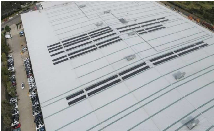
Eastern Creek Distribution Center in Sydney, Australia
